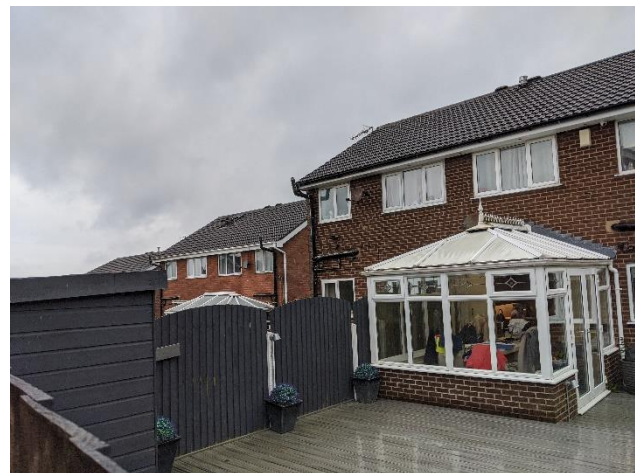
Photo 4: Part of rear elevation of no. 55 (right), with no. 53 adjoining (left)
