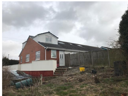
Photo 2: rear elevation and existing dormer
