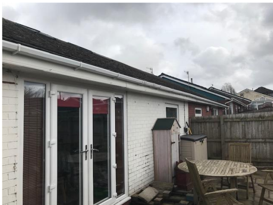
Photo 3: existing rear elevation
