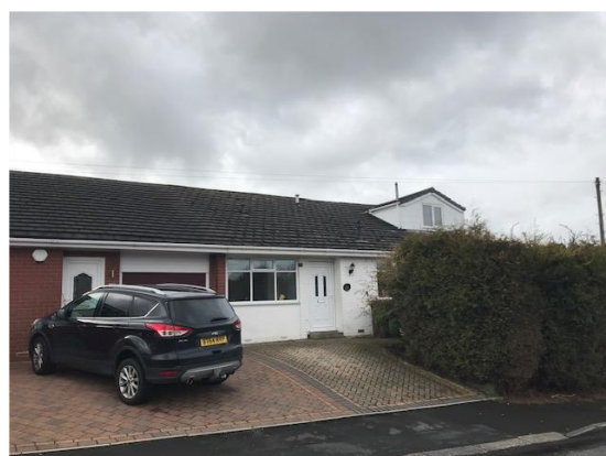
Photo 4: existing front elevation
