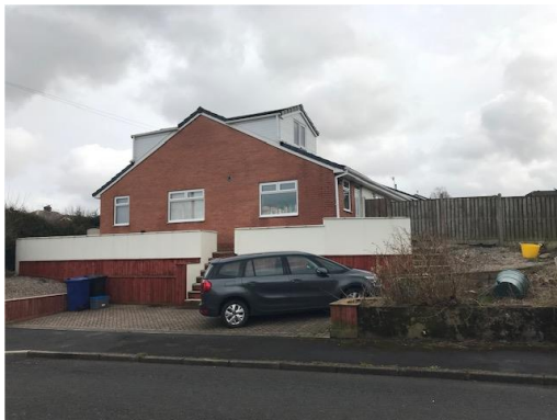
Photo 1: gable elevation from Micklehurst Crescent
